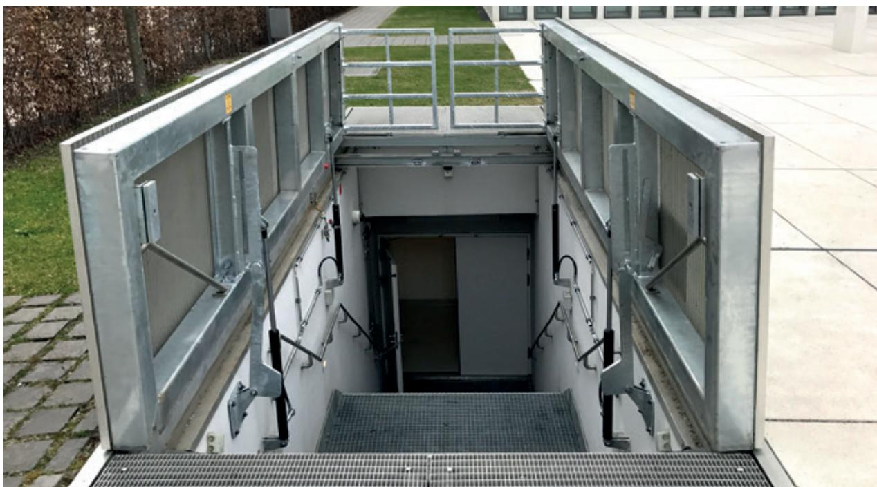
2-piece floor hatch as an emergency exit, Munich
