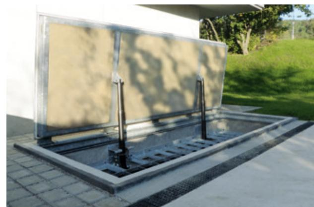
Hydraulic cover on a woodchip silo with a fire protection classification of F90,
