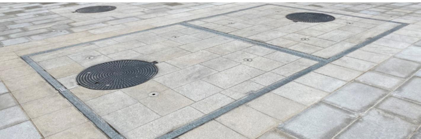
Underground railway station with entry and exit openings for smoke extraction technology and inspection openings for quick access,
