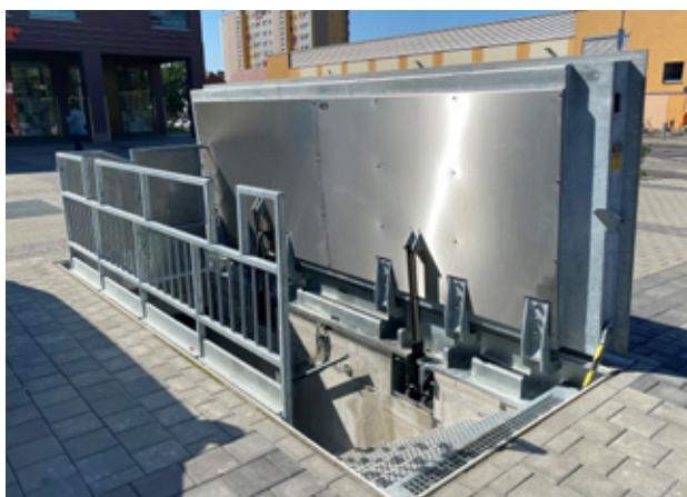
Hydraulic escape hatch with collapse protection, Berlin
