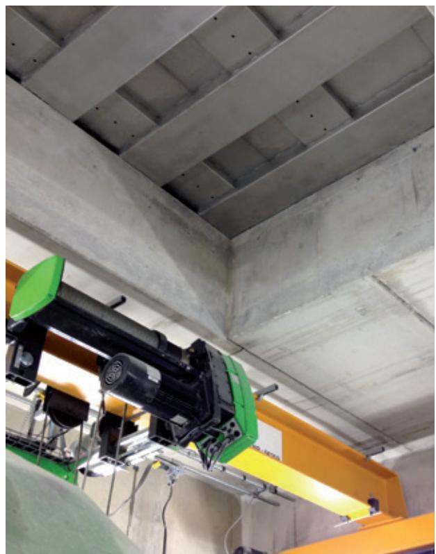
View from below of a floodproof cover on an assembly opening,
