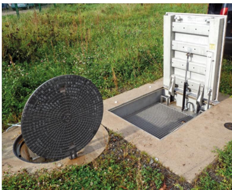
Combination: round cast-iron cover with hinge
