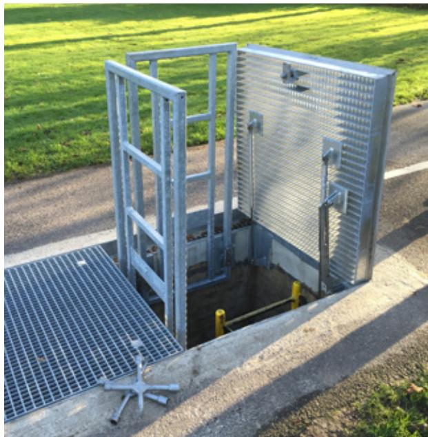
Escape hatch with a telescopically retractable grating, Leverkusen
