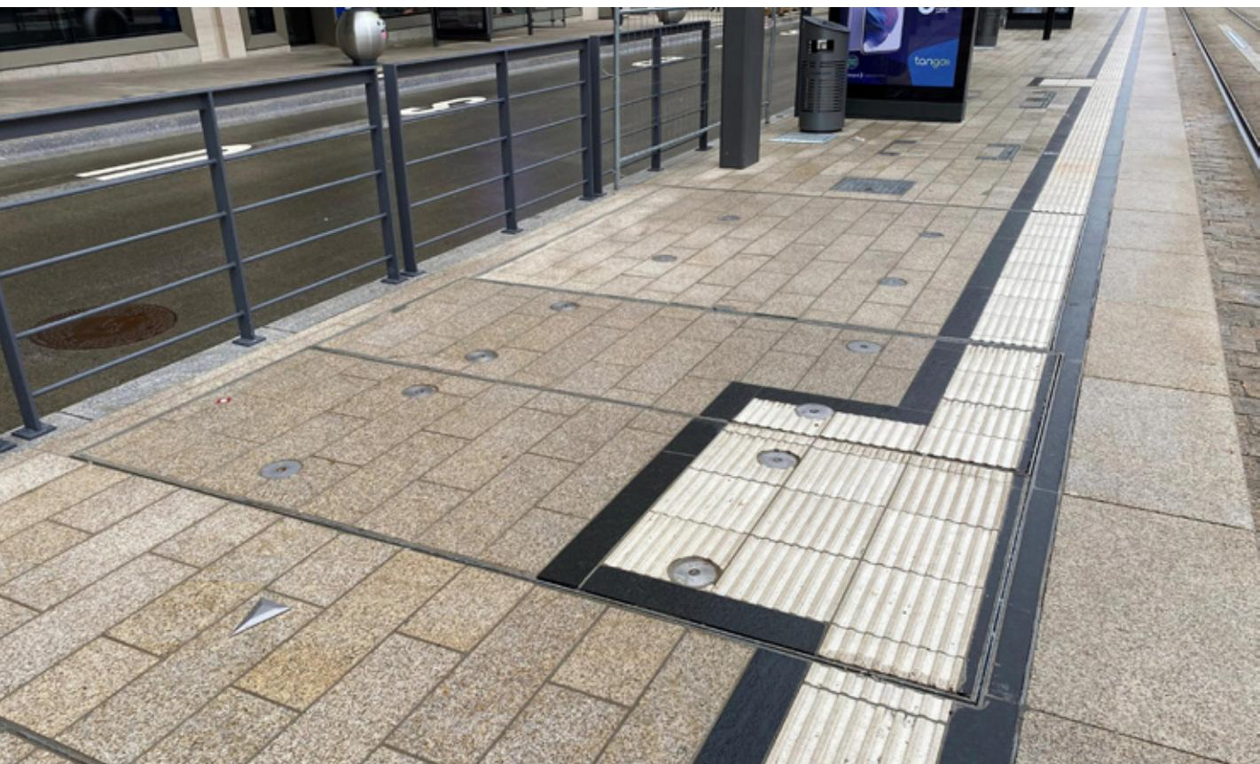
Discreet, as little metal on the surface as possible – this can be realised with pavable floor hatches, Luxembourg
