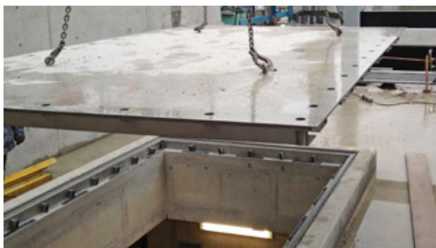
View from below of a floodproof cover on an assembly opening,
